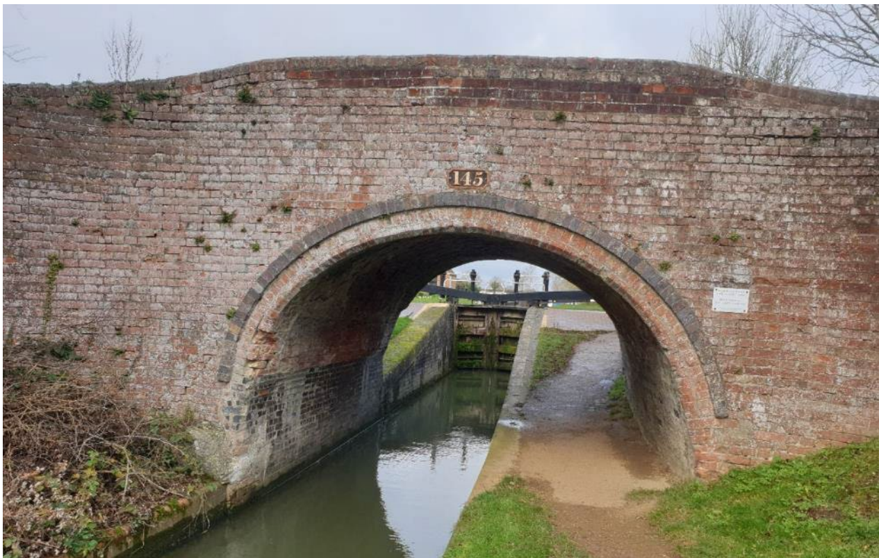
Figure 2-6: South elevation of Claydon Canal Bridge [2021].
