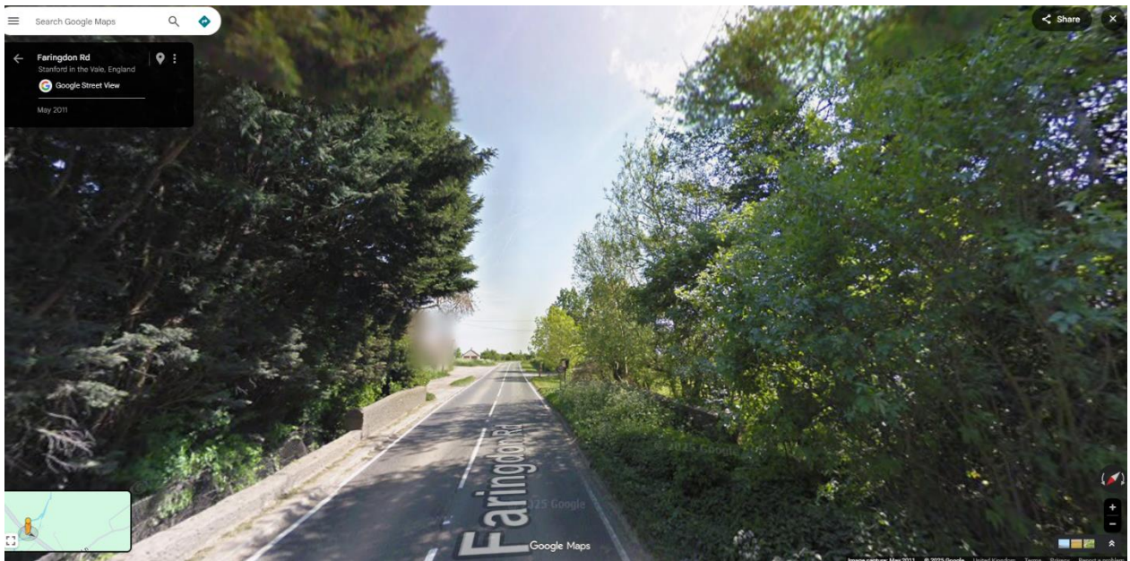
Bridge over the river Ock with very narrow pavement
