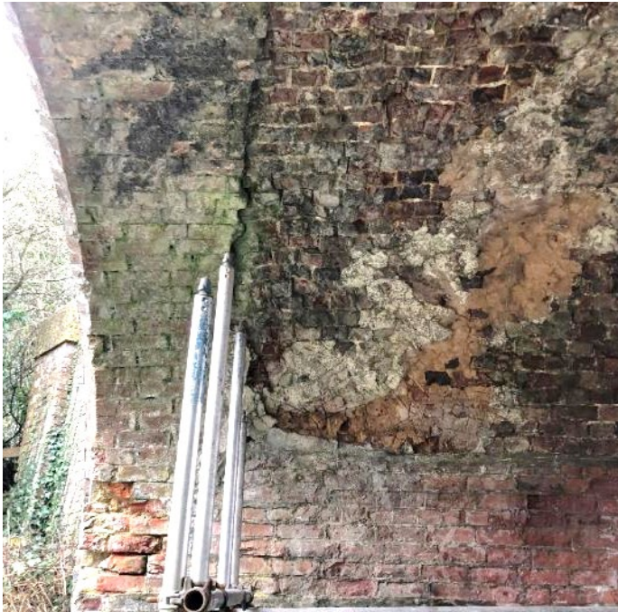
Figure 2-4: South end of arch barrel [2024].
